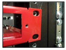
Determine the location on the rack that the taps are to be installed. Line up the mounting holes on each side of the rack mount with the holes on the rack.
